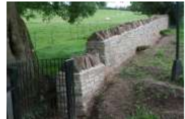
The re-built churchyard wall
